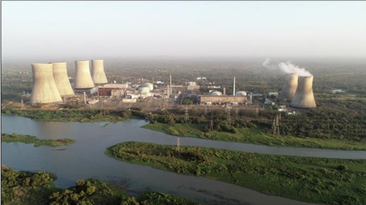
Kakrapar Atomic Power Station – Site view
