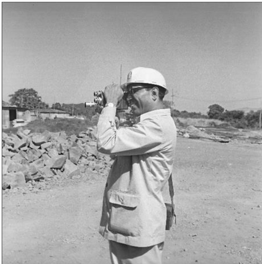
Dr Homi Bhabha during the construction phase of AEET
